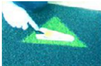
Ensure granules are level and in line with existing surface
